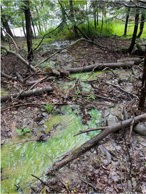
#12: D5-1 / Aug 15, 2023. Looking downstream, Burden Lake in background. Note debris obstructing the drainage course.
