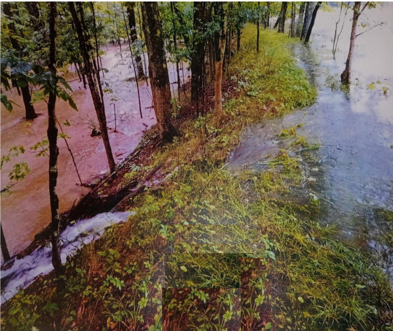
Water flowing over the berm (canal to the right). Photo taken during flood of 2021.
