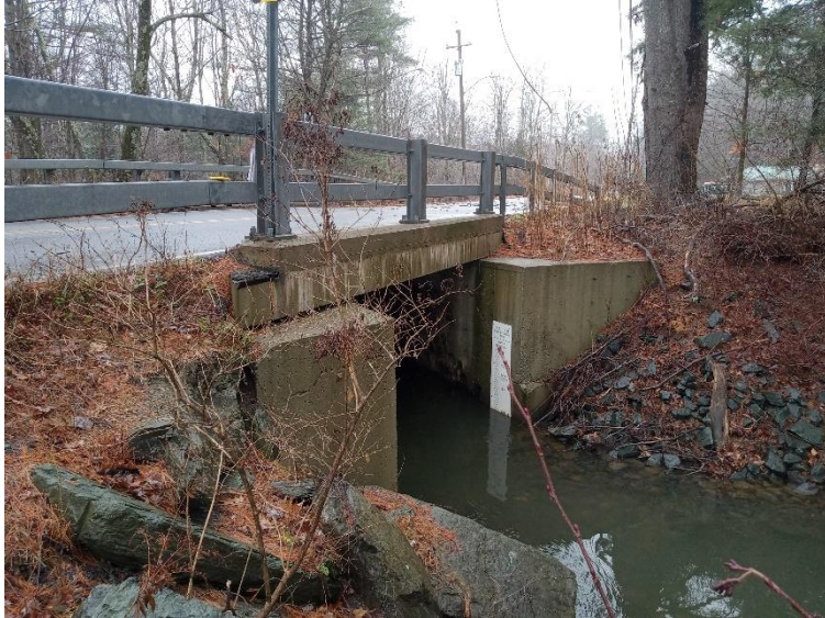
Lake side of Spillway
