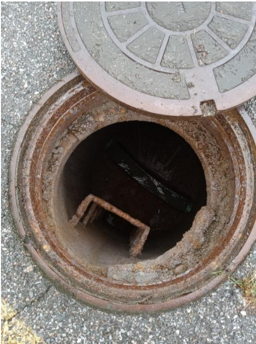
Sewer manhole at least 10' deep.
