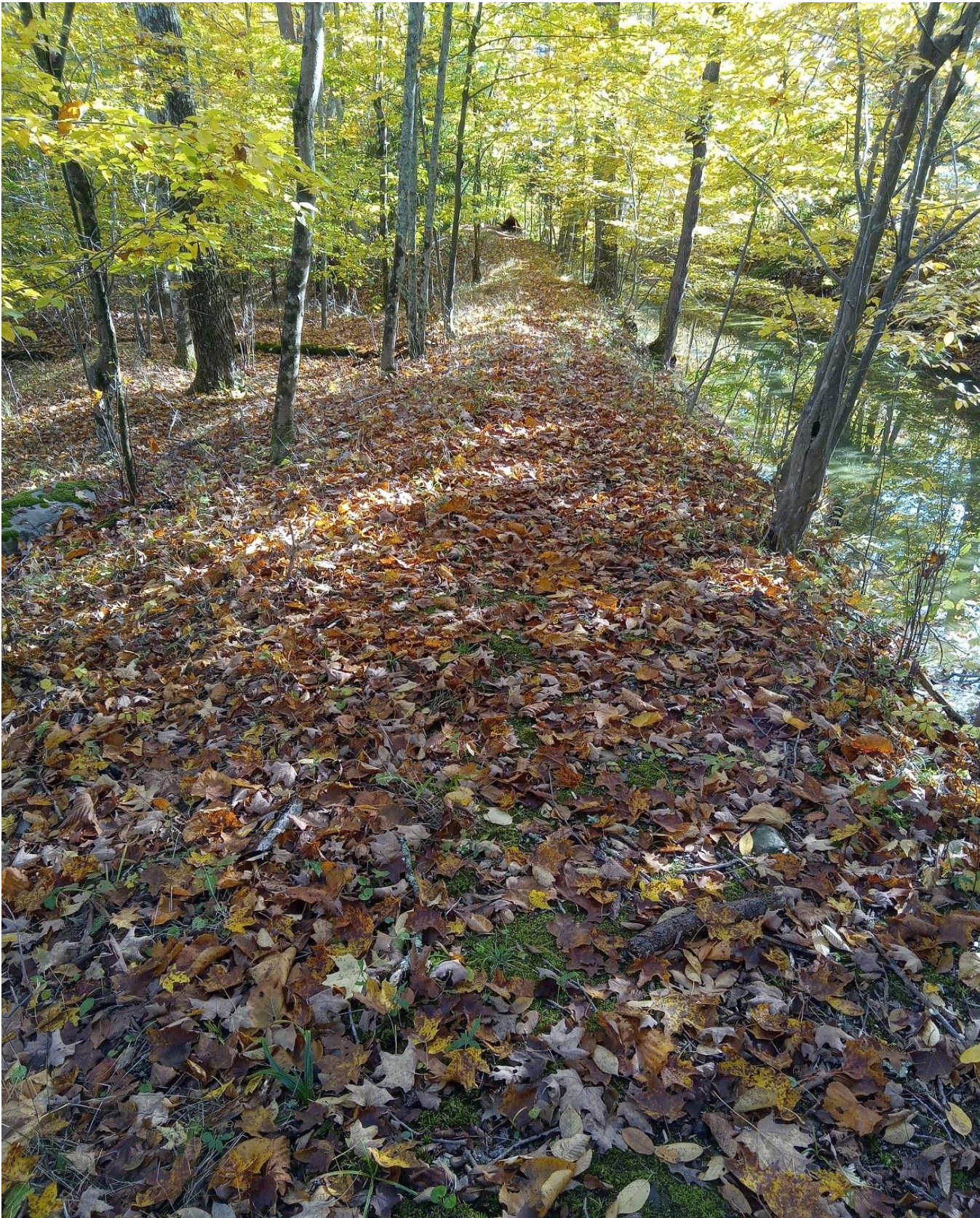
Berm after the flood, with canal to right.
