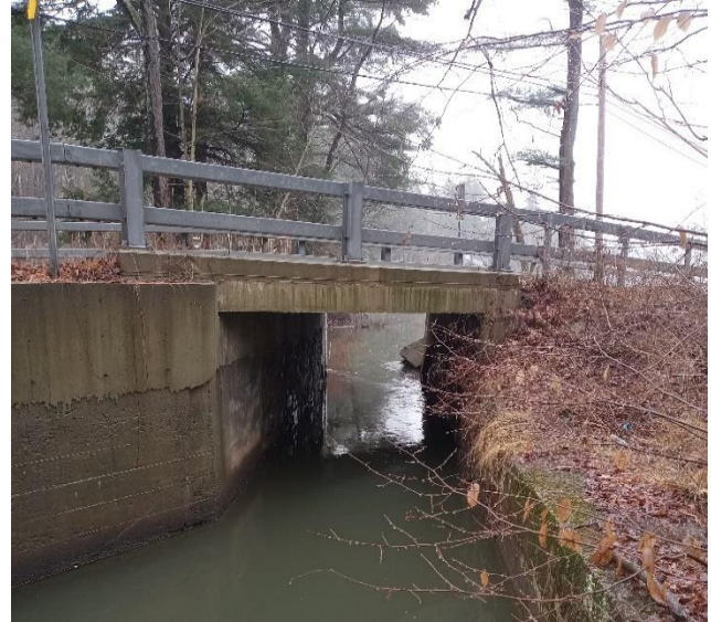
Canal side of Spillway
