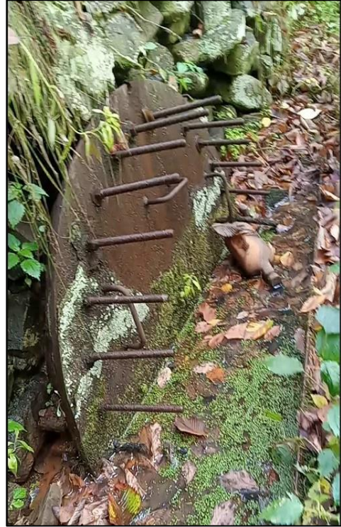
30" pipe capped off
